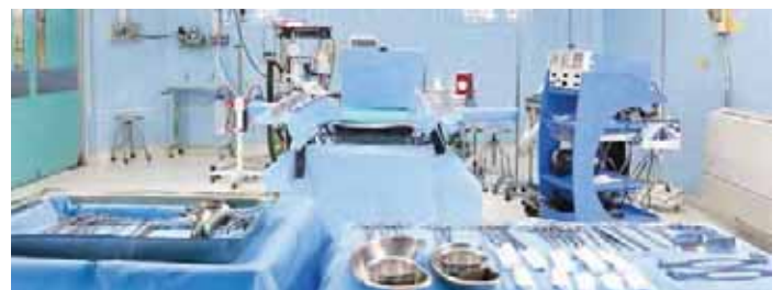
Figure 3. Modular clean room
